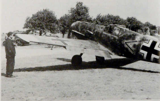
BELOW: Displaying its yellow wing tip to advantage, the same aircraft is seen leaving its dispersal. The upper surfaces of the wings retain the 02/71 camouflaze while the fuselage finish is a fairly densely applied green mottle over an irregular misting of 02.
