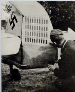
ABOVE: Major Galland's Bf 109 E-4/N, W.Nr. 5819, possibly photographed at Le Touquet in 1941. The fresh paint beneath the forward Stab symbols is believed to indicate the recent installation of nitrous oxide equipment to increase engine power.
