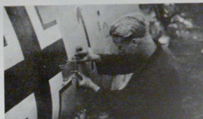
ABOVE: Provided no part of the internal aircraft structure was weakened, simple battle damage could be repaired in the field. Here a member of the ground staff patches bullet holes in the fuselage of a Bf 109; 26 Bf 109s at Cañiers.
