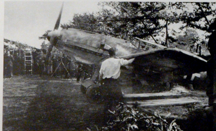
LEFT: A Bf 109 E-3, believed to be from 3./ Freize Jagdgruppe 210 at Denzin, taxis from its camouflaged dispersal. The two wooden planks prevented the main undercarriage wheels from sinking into the soft earth.
